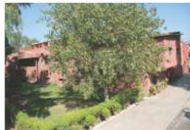
Paramount Blades Factory
